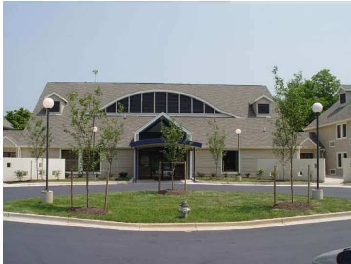
Seneca Heights Supportive Housing Gaithersburg, Montgomery County PRHP Loan
